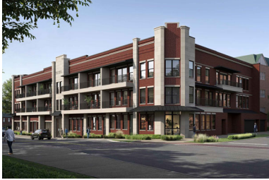
NORTHEAST CORNER LOOKING SOUTH
