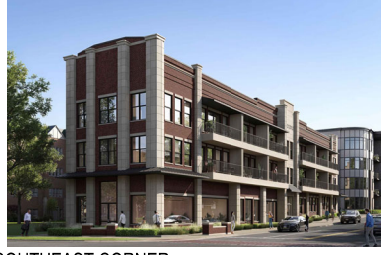
SOUTHEAST CORNER LOOKING NORTH
